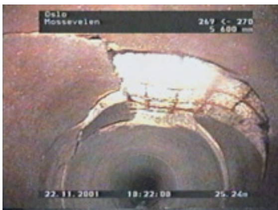
Reparert hull.
